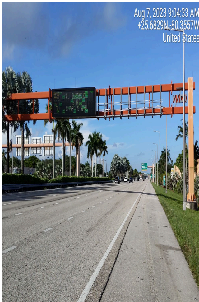
DETERIORATED PAINT ON OVERHEAD SIGN (STRUCTURE # 87A327)
