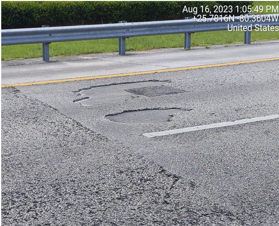
DETERIORATED ASPHALT
