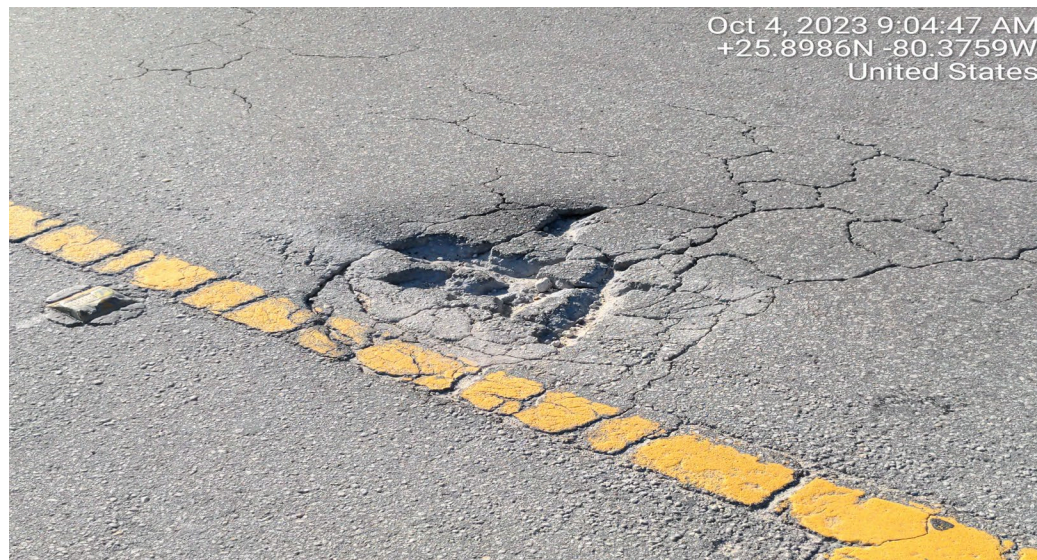
DETERIORATED STRIPING AND POTHOLE
