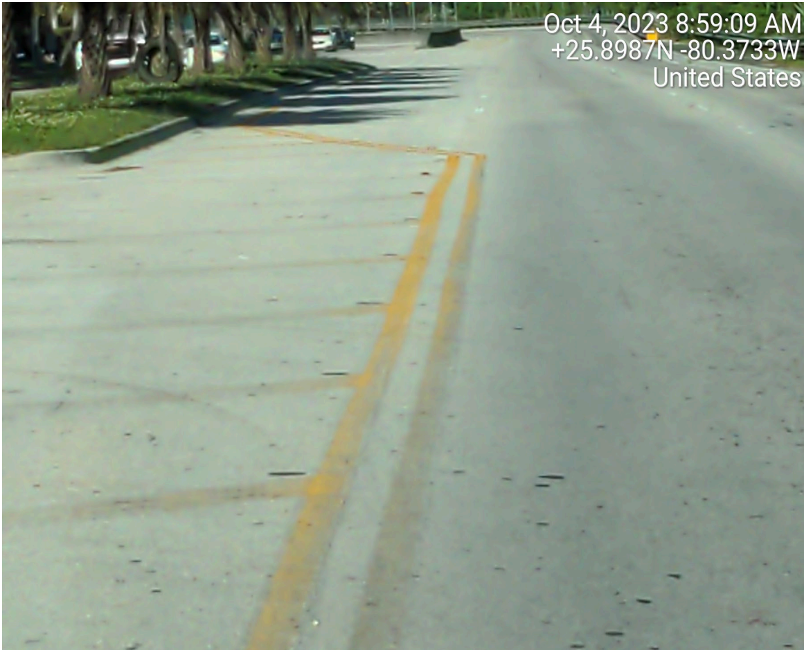
DETERIORATED STRIPING IN GORE AREA
