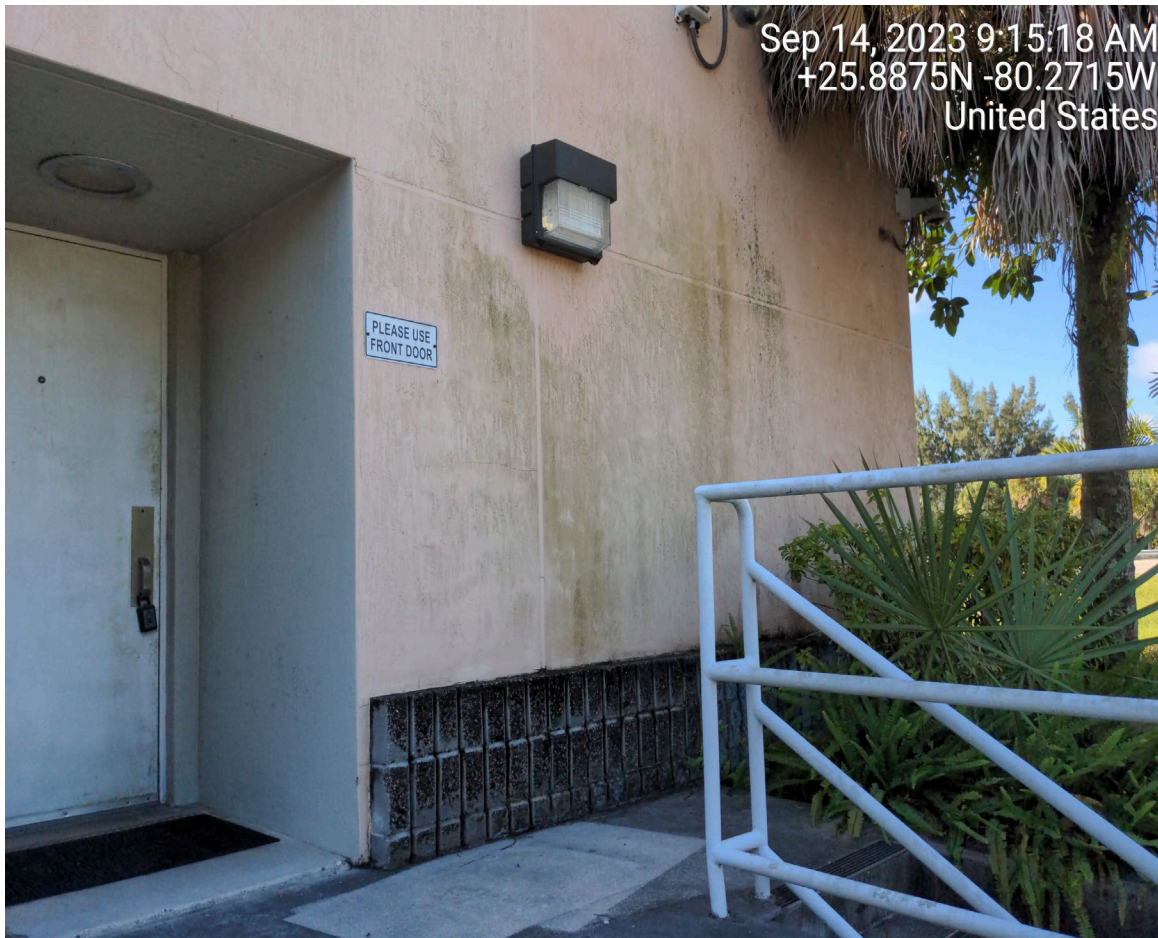
MOLD STAINS ON EXTERIOR WALLS
