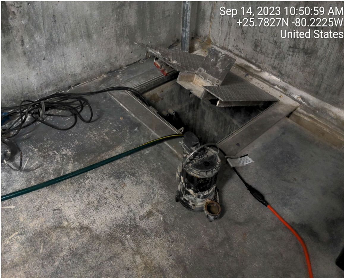
DAMAGED SUMP PUMP
