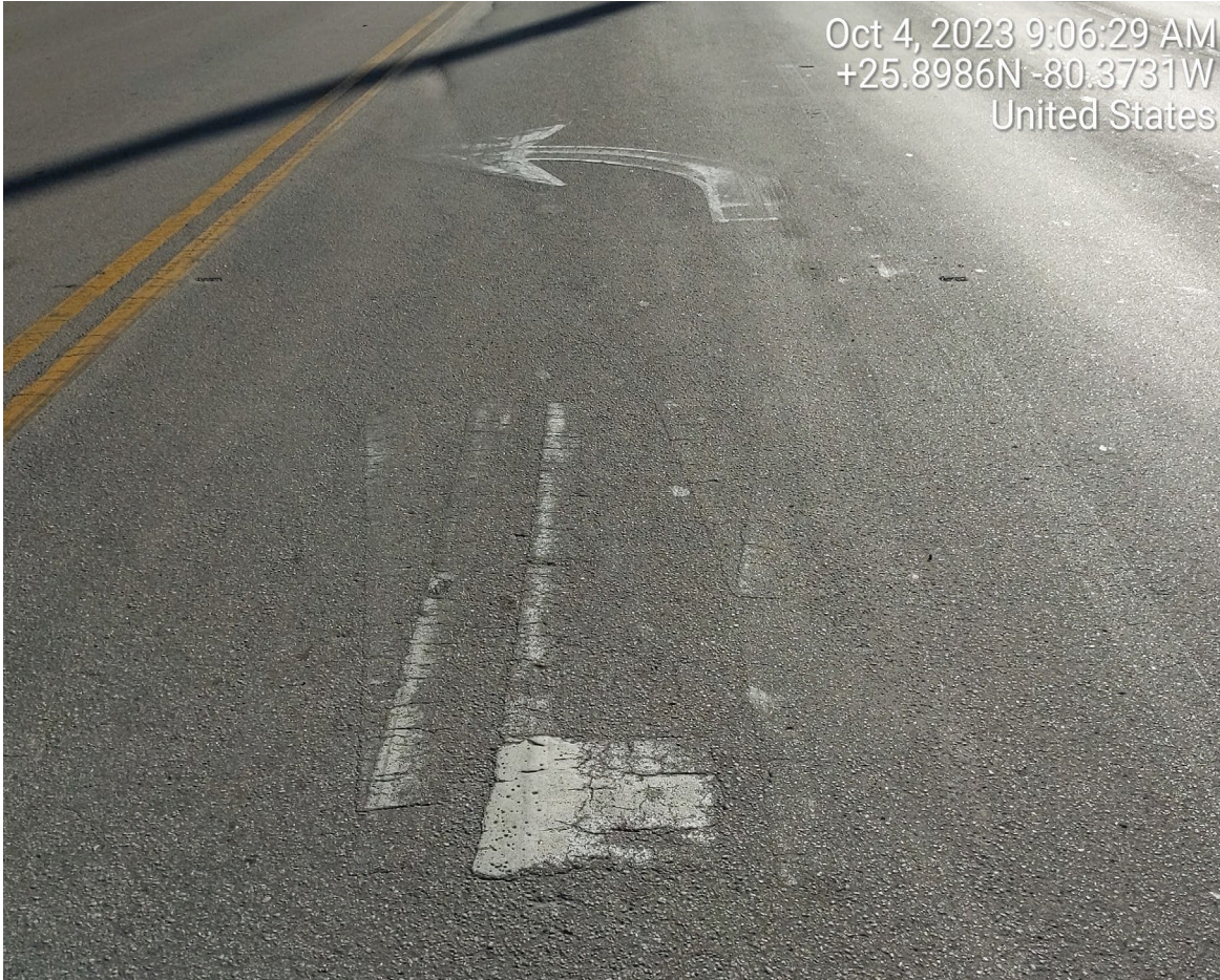
DETERIORATED PAVEMENT MESSAGE AND TURN ARROW
