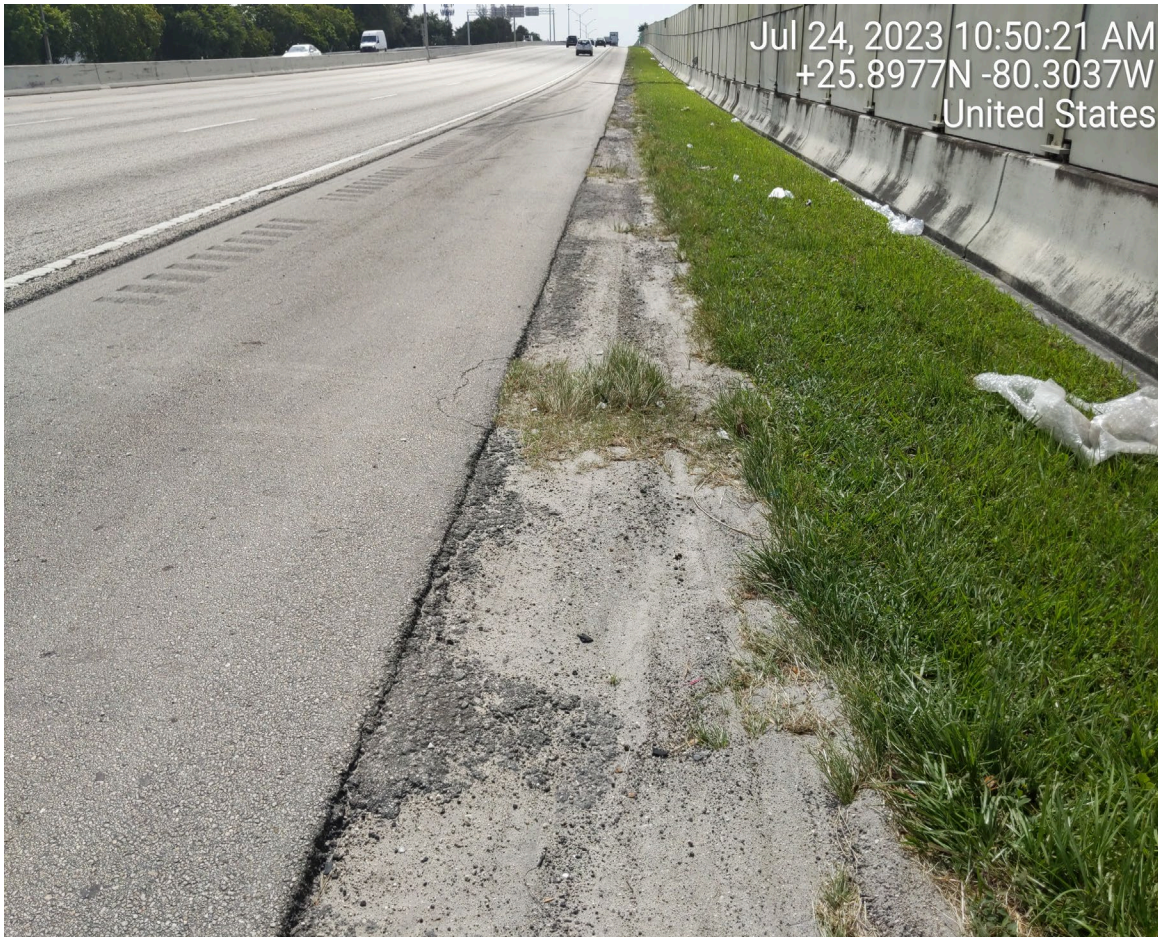
SHOULDER DROP OFF AND MISSING TURF
