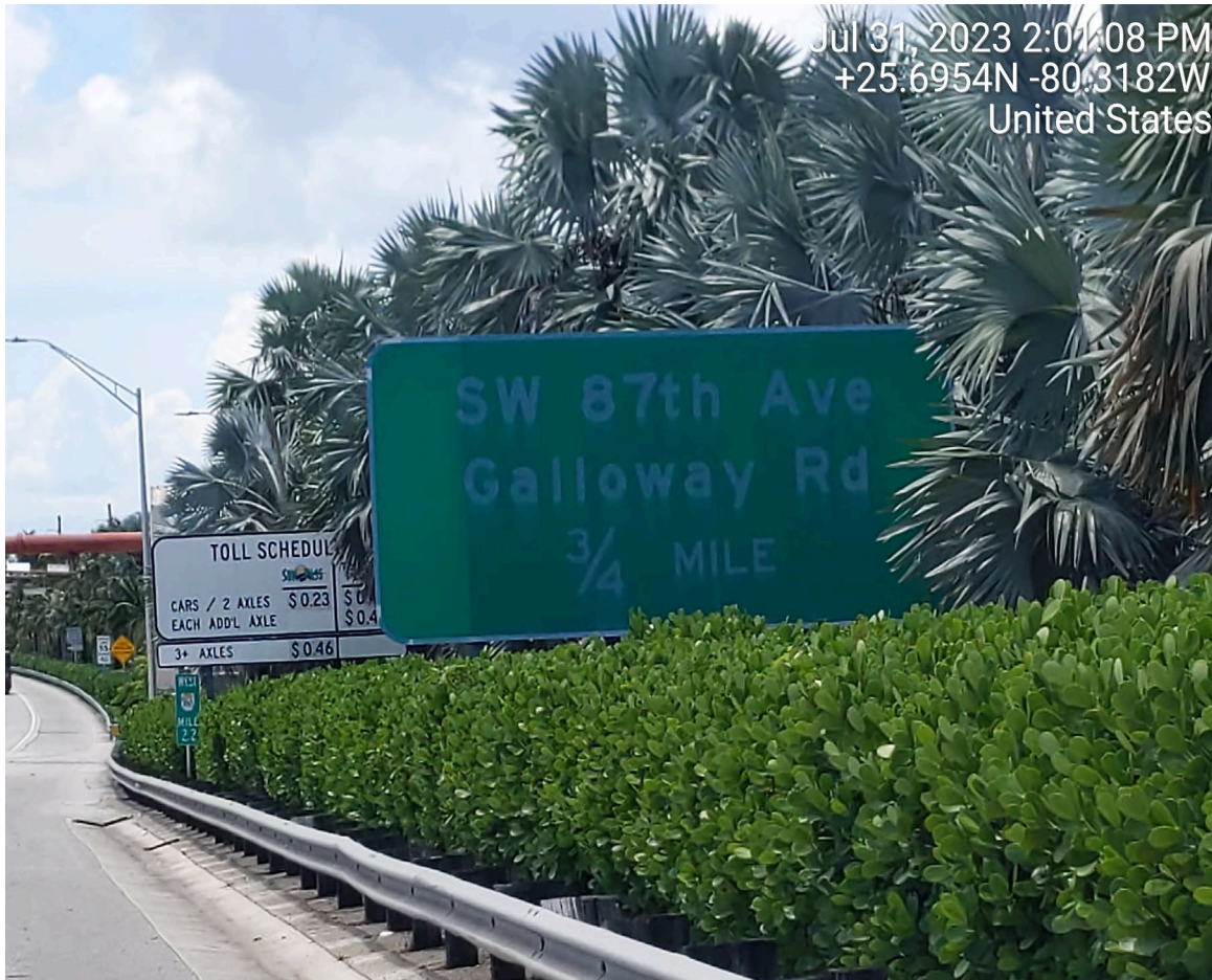
DETERIORATED REFLECTIVE SHEETING
