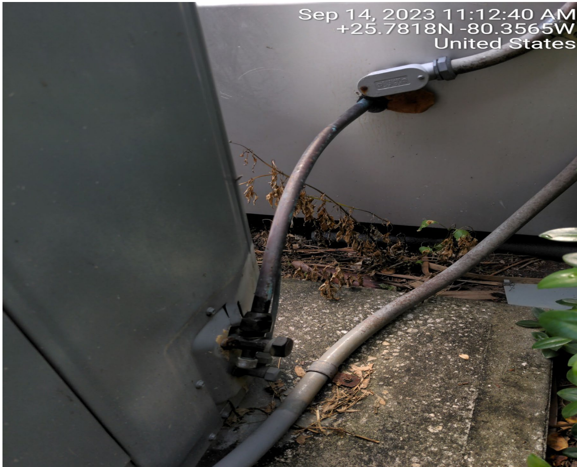
MISSING INSULATION ON HVAC REFRIGERANT LINE
