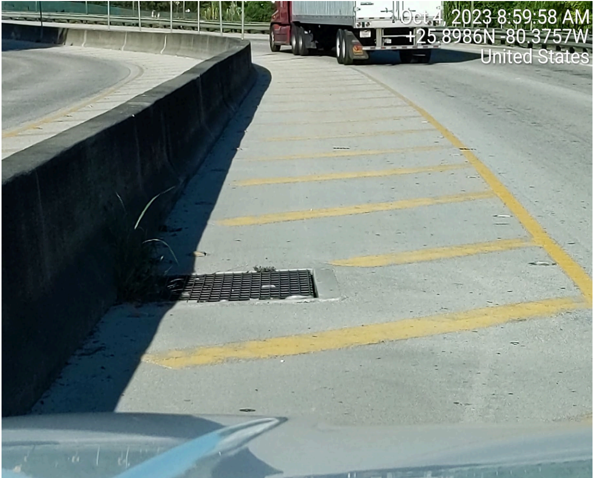
SILTED DRAINAGE INLET (TYPICAL AT VARIOUS LOCATIONS)
