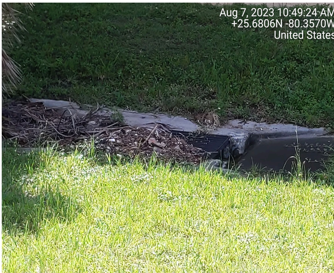
DEBRIS ON DRAINAGE STRUCTURE
