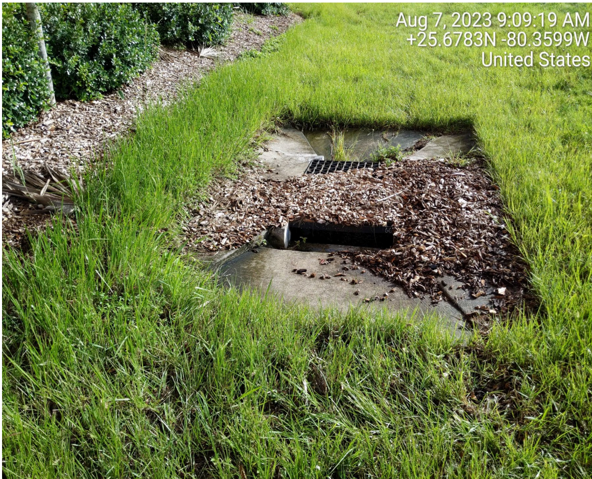
MULCH OBSTRUCTING STORM DRAIN
