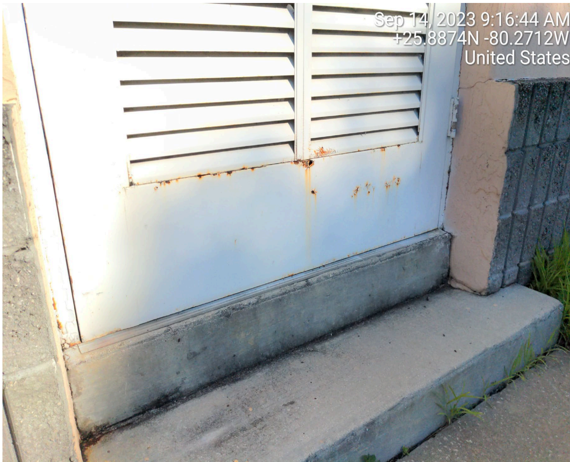
SURFACE CORROSION ON METAL DOOR
