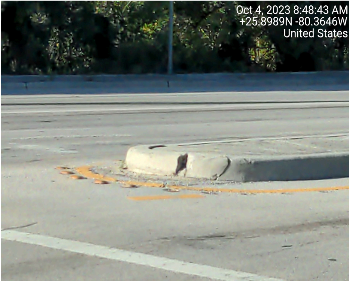
DAMAGED TRAFFIC SEPATATOR
