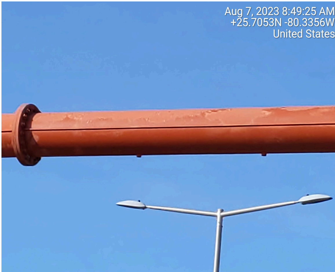
DETERIORATED PAINT ON MONOTUBE (STRUCTURE # 87A131)
