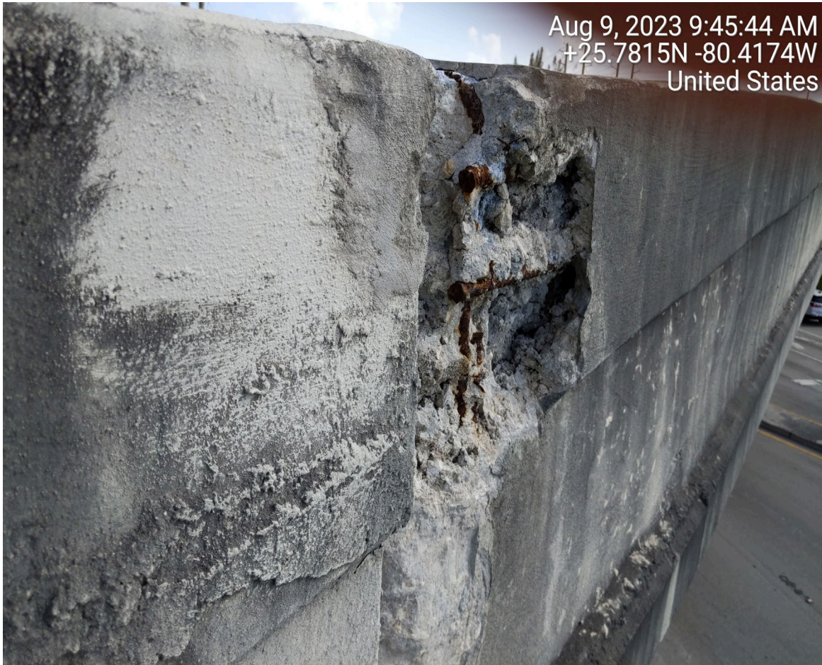
SPALL ON EXTERIOR FACE OF TRAFFIC RAILING AT ABUTMENT 1 BRIDGE NO. 870966
