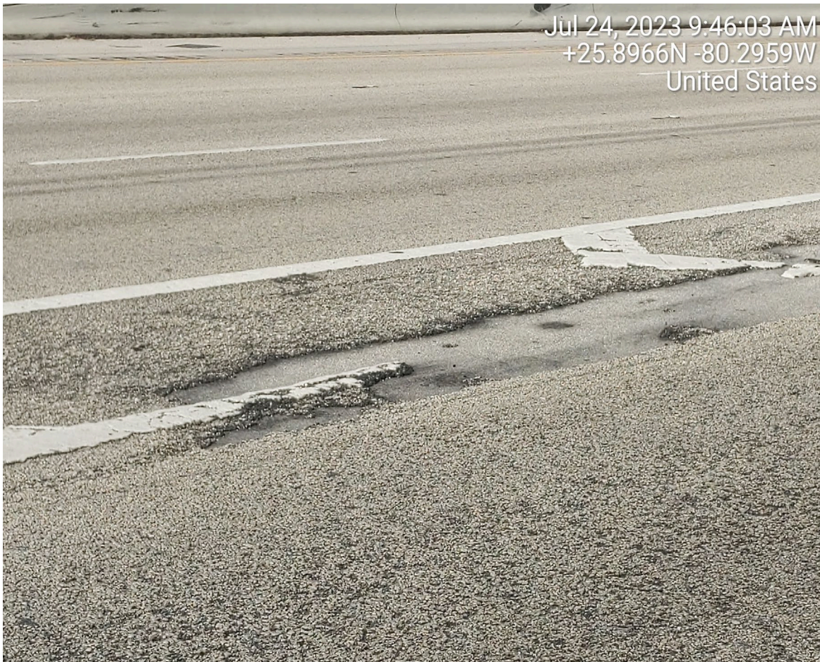
DETERIORATED ASPHALT PAVEMENT
