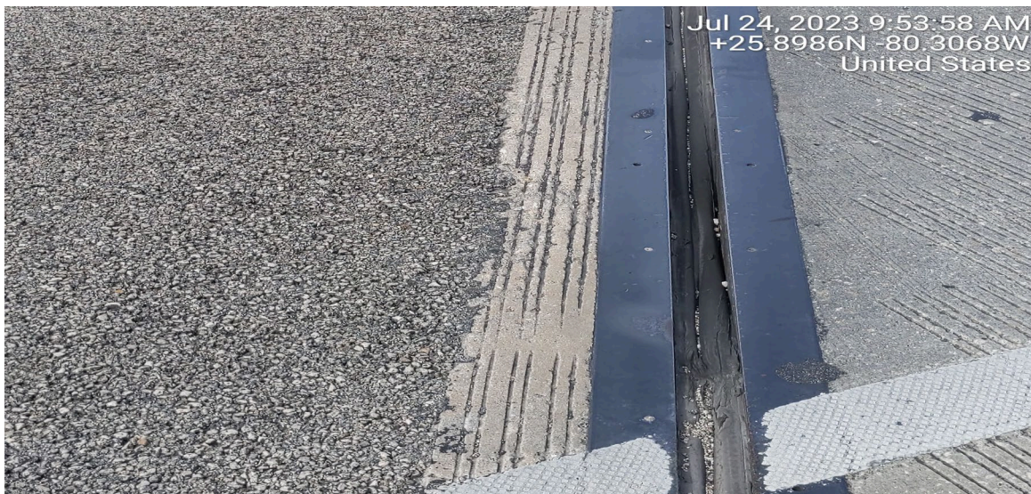
DAMAGED BRIDGE EXPANSION JOINT (BRIDGE # 870708)
