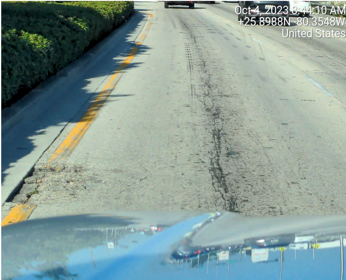
POTHOLE ON INSIDE LANE AND DETERIORATED STRIPING
