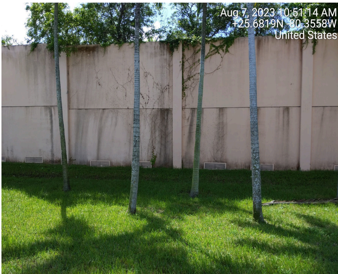
DETERIORATED CLASS V COATING ON SOUND WALL
