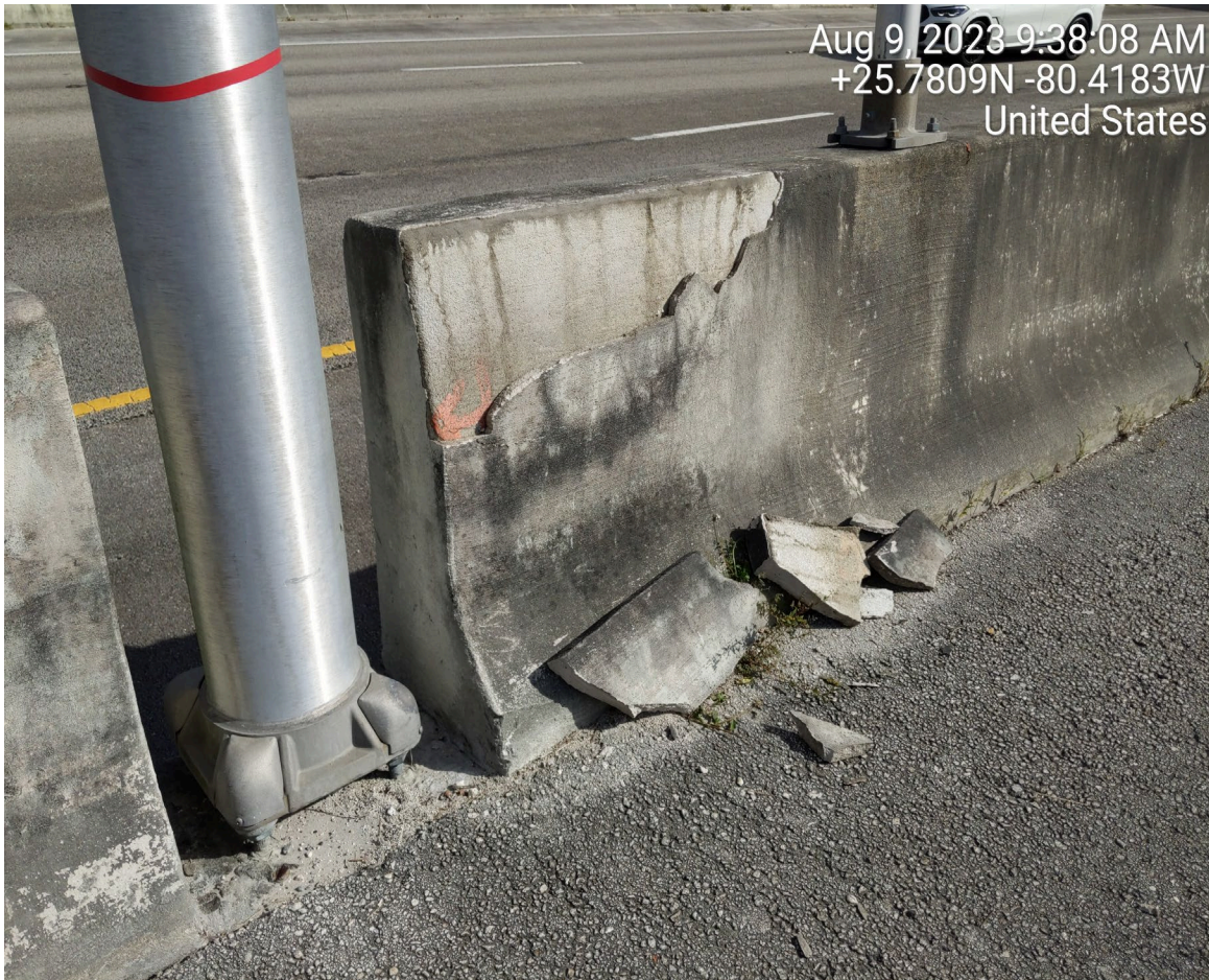
SPALL ON BARRIER WALL
