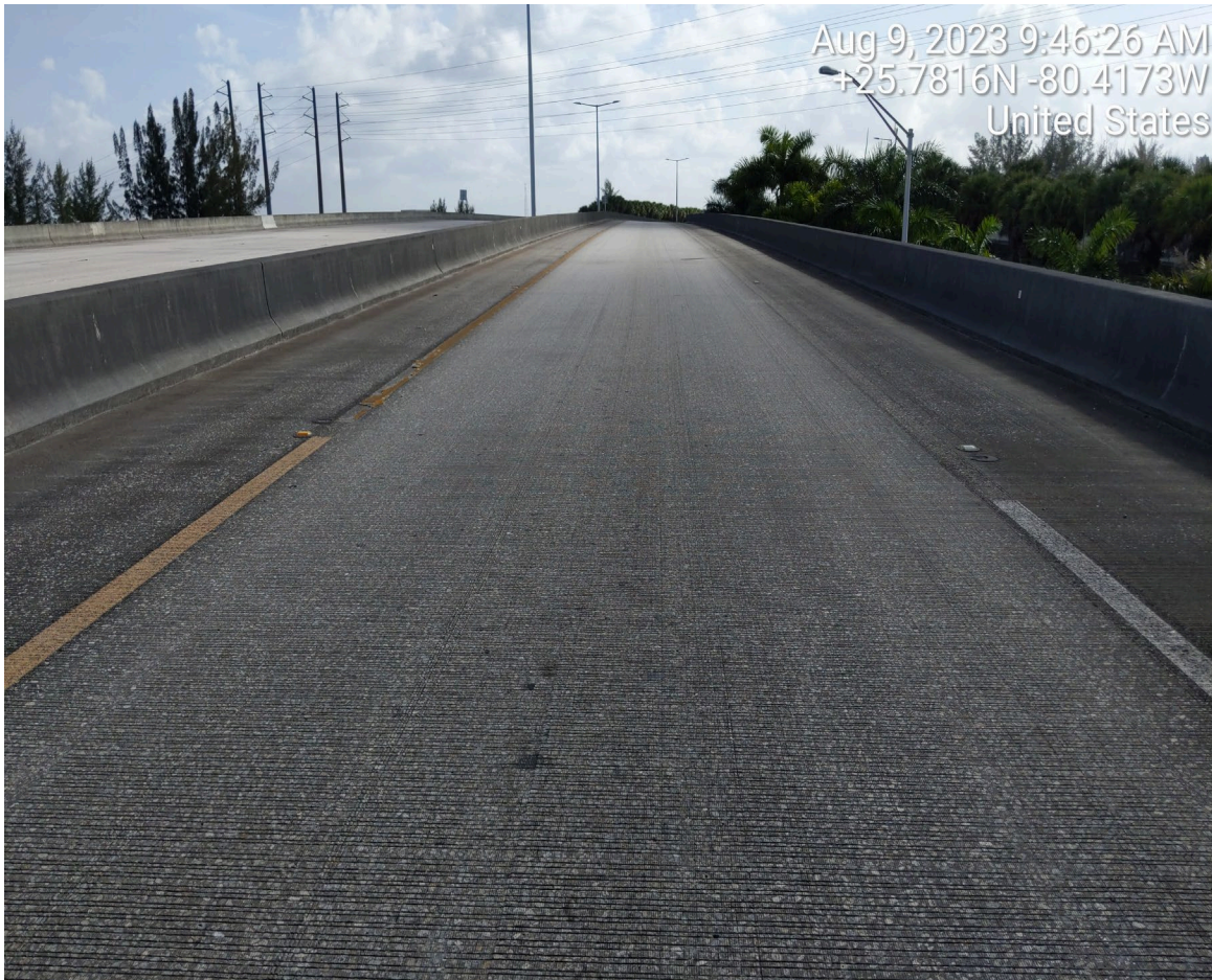
DETERIORATED STRIPING (BRIDGE No. 871008)
