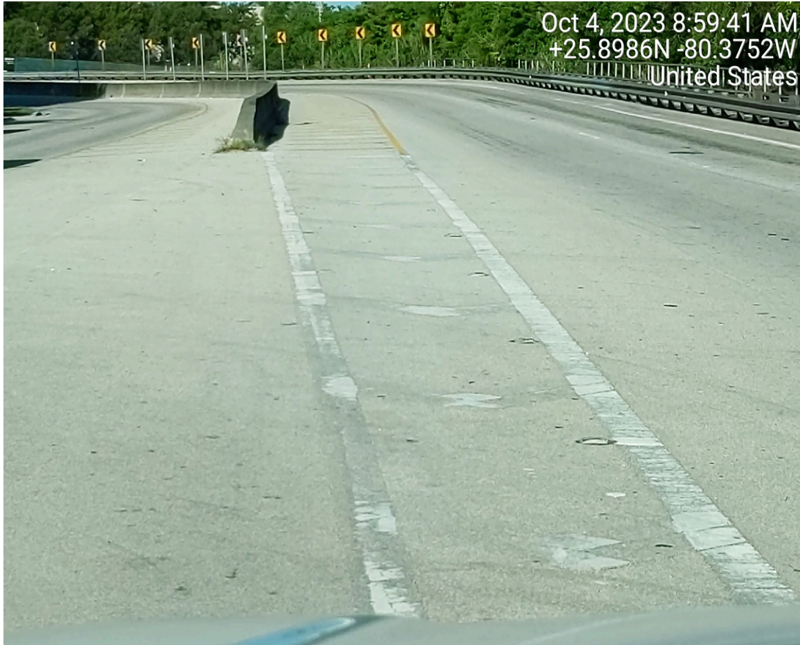
DETERIORATED STRIPING IN GORE AREA
