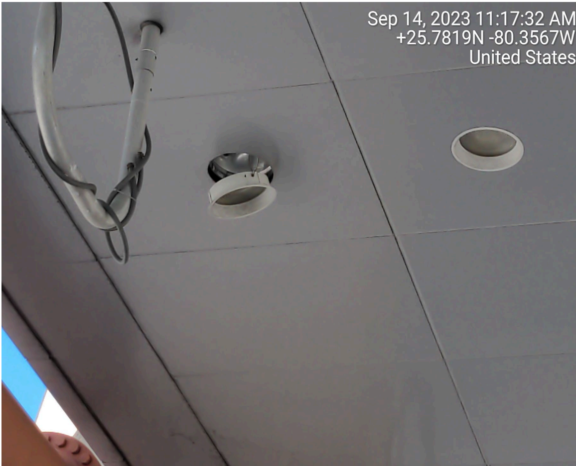
HANGING RECESSED LUMINAIRE COVER
