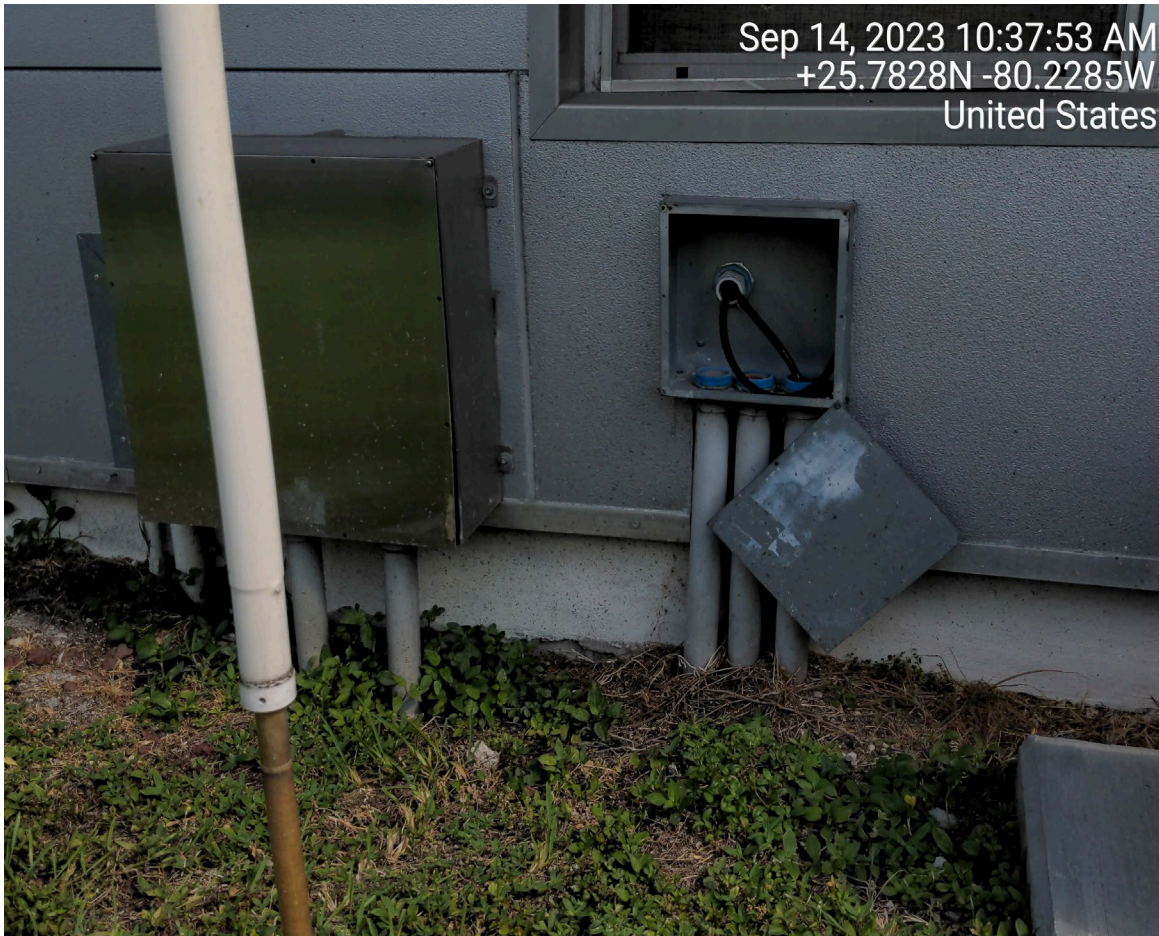
LOOSE PULL BOX COVER PLATE
