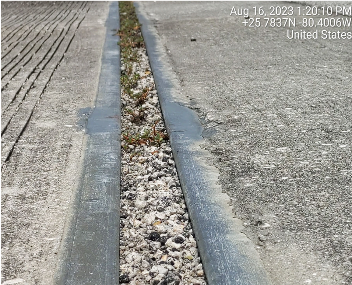
SEDIMENT AND DEBRIS ACCUMULATED ON BRIDGE EXPANSION JOINTS (BRIDGE No. 871002)
