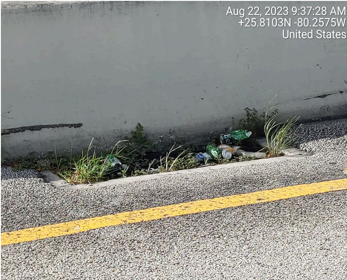
SILTED DRAINAGE STRUCTURE
