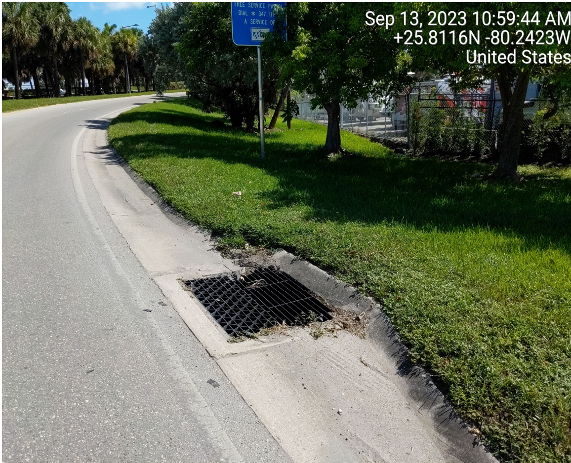
SILTED DRAINAGE STRUCTURE (TYPICAL AT VARIOUS LOCATIONS)
