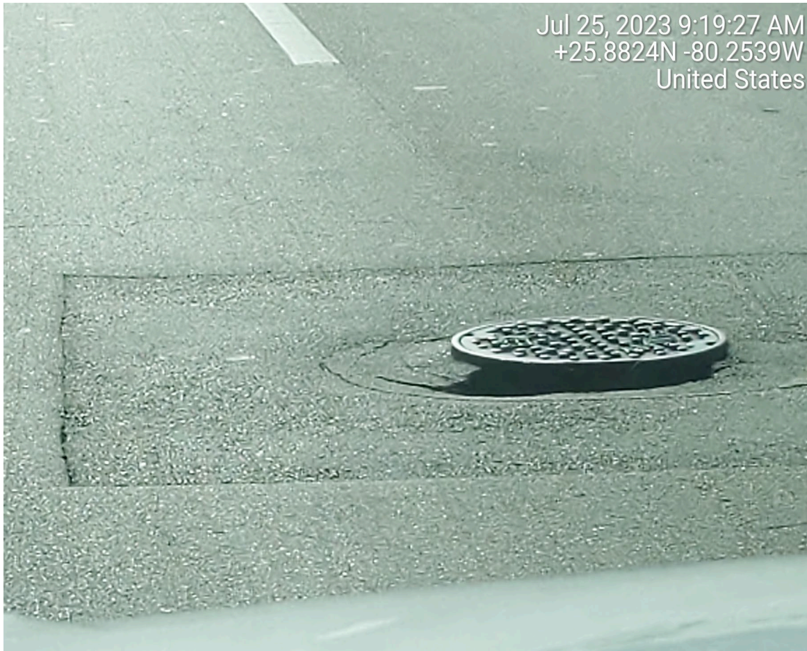
DAMAGED MANHOLE AND DETERIORATED PAVEMENT
