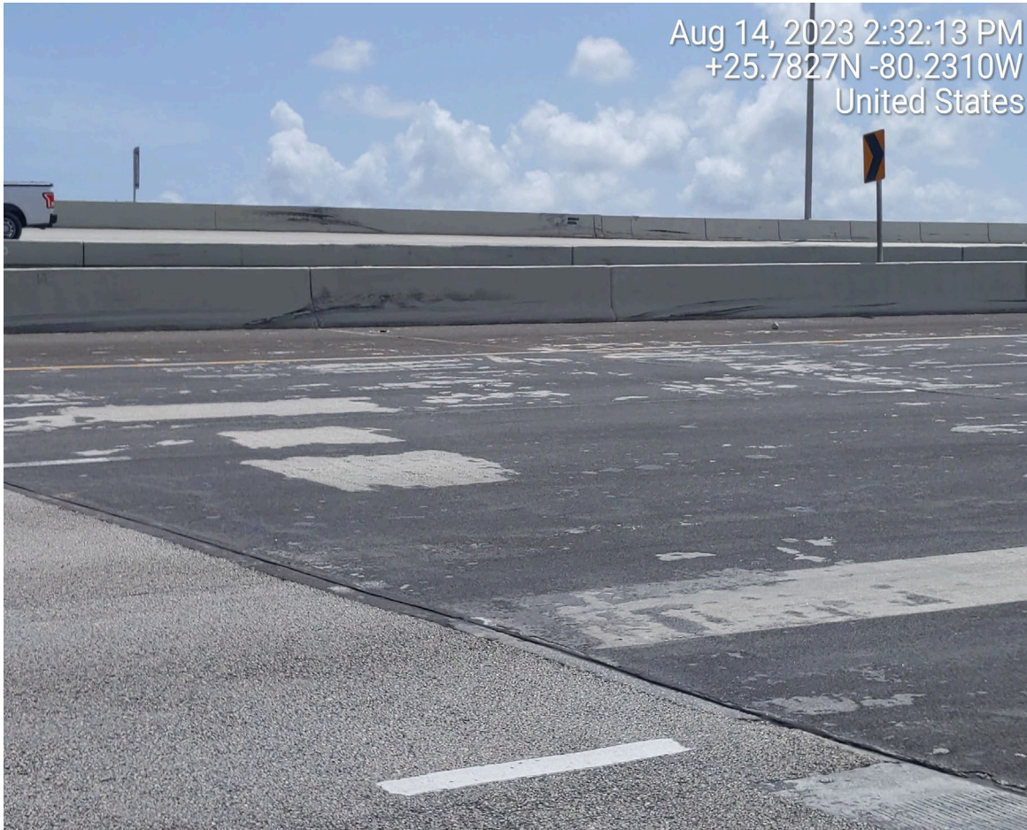
DETERIORATED DECK OVERLAY (BRIDGE # 870145)
