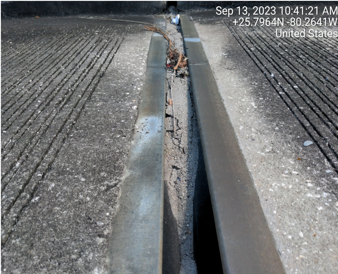
SILT AND DEBRIS ON BRIDGE JOINTS (TYPICAL AT VARIOUS LOCATIONS) BRIDGE No. 870725
