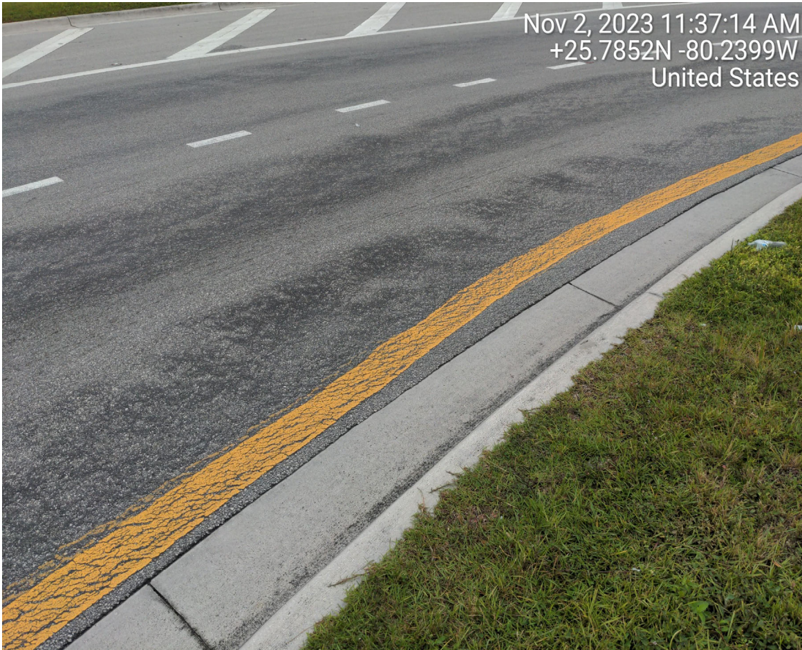
DAMAGED PAVEMENT DUE TO SETTLEMENT
