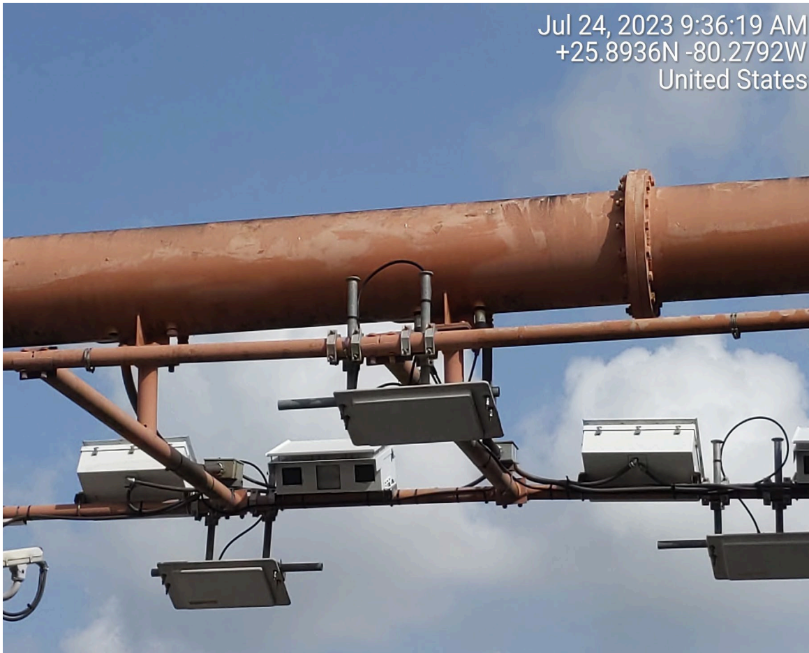
DETERIORATED PAINT ON ORT MONOTUBE (STRUCTURE # 87S932)
