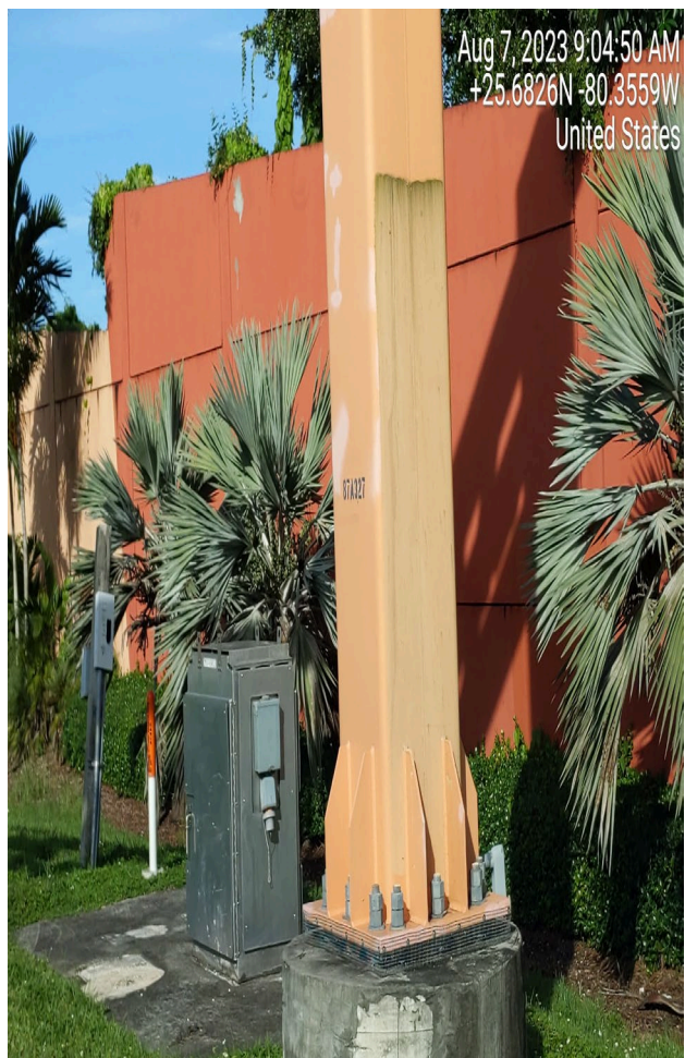
DETERIORATED PAINT ON OVERHEAD SIGN (STRUCTURE # 87A327)
