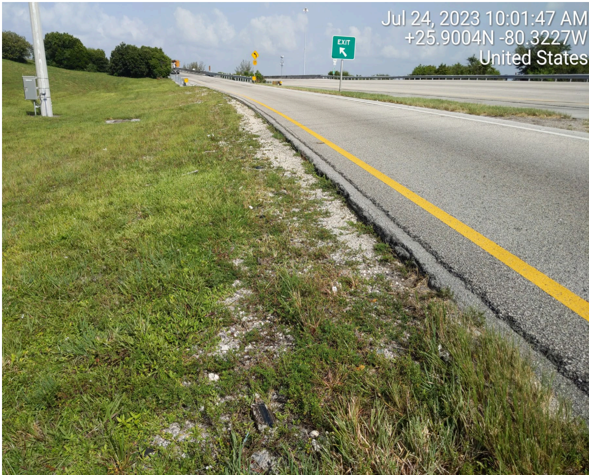
SHOULDER DROP OFF AND MISSING TURF
