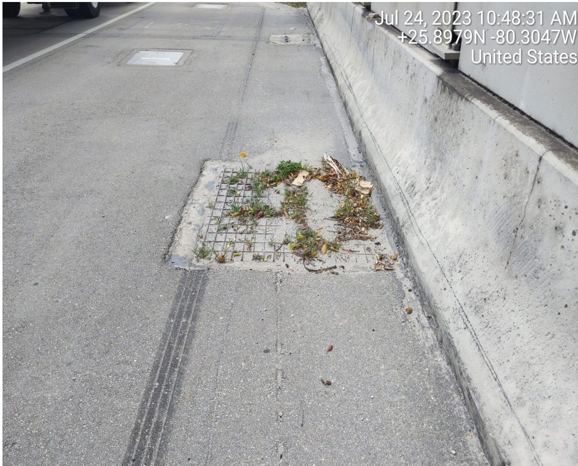
SILTED DRAINAGE STRUCTURE (TYPICAL AT VARIOUS LOCATIONS)
