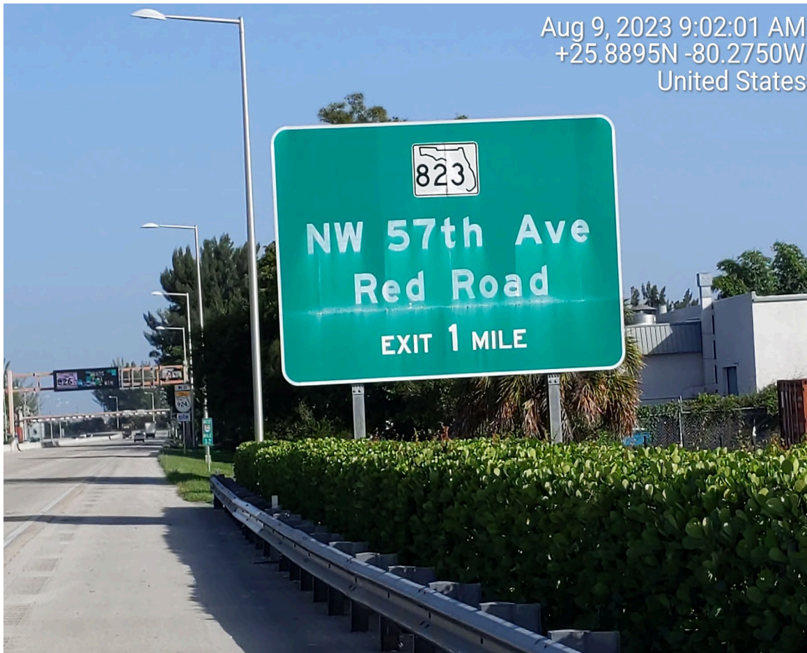
DETERIORATED REFLECTIVE SHEETING
