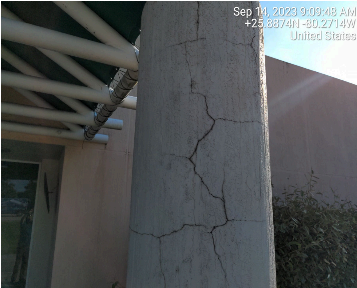
CRACKS ON COLUMN
