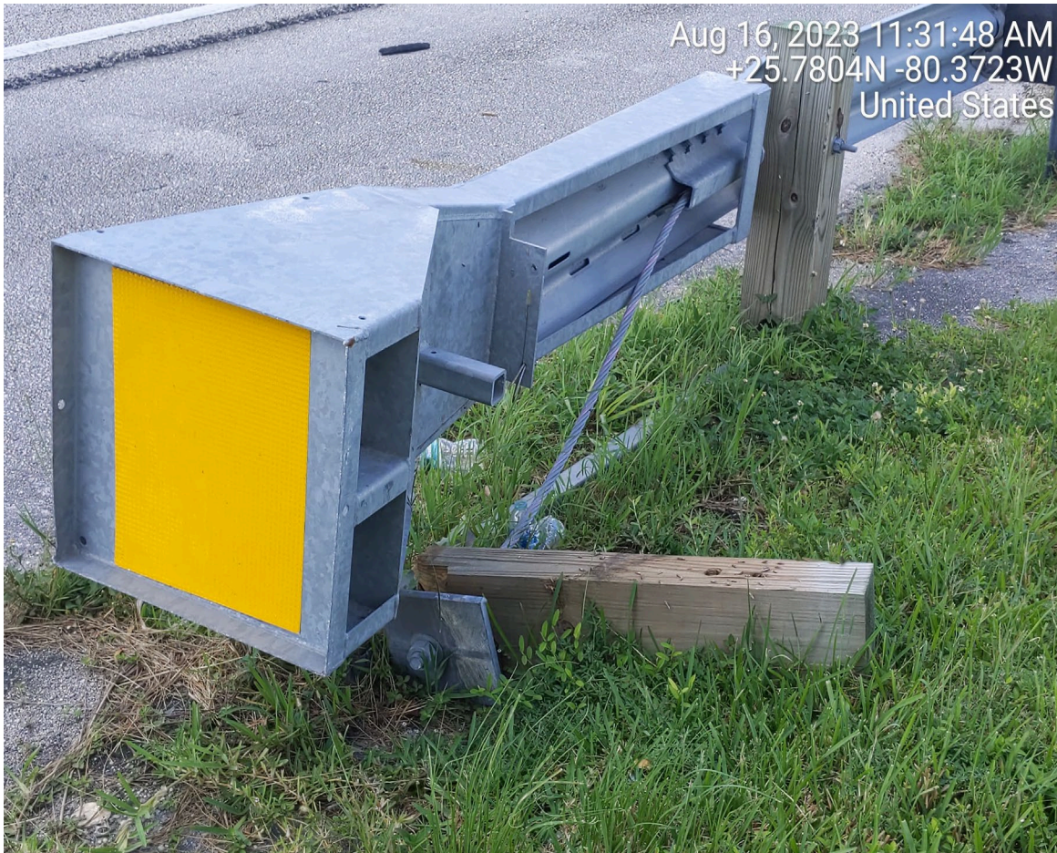
DAMAGED POST ON END TREATMENT
