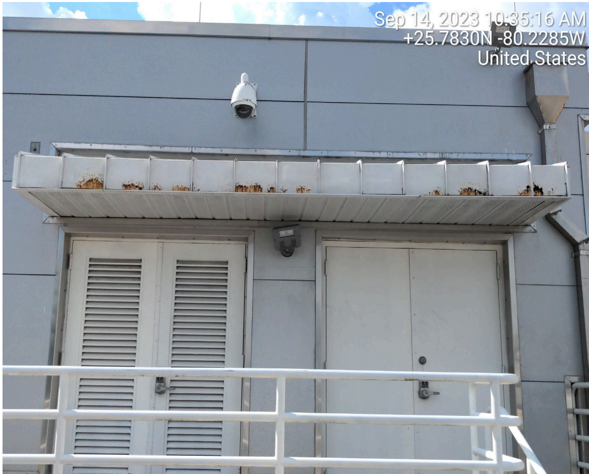
SURFACE CORROSION ON METAL AWNING
