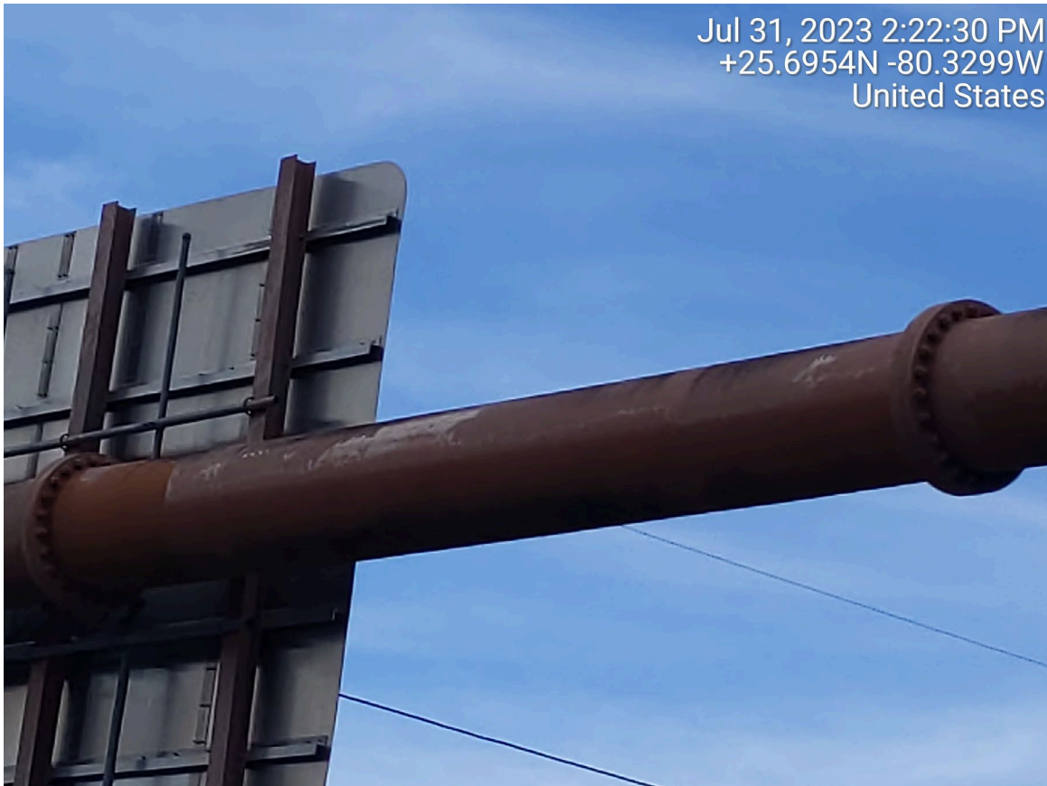
DETERIORATED PAINT ON MONOTUBE
