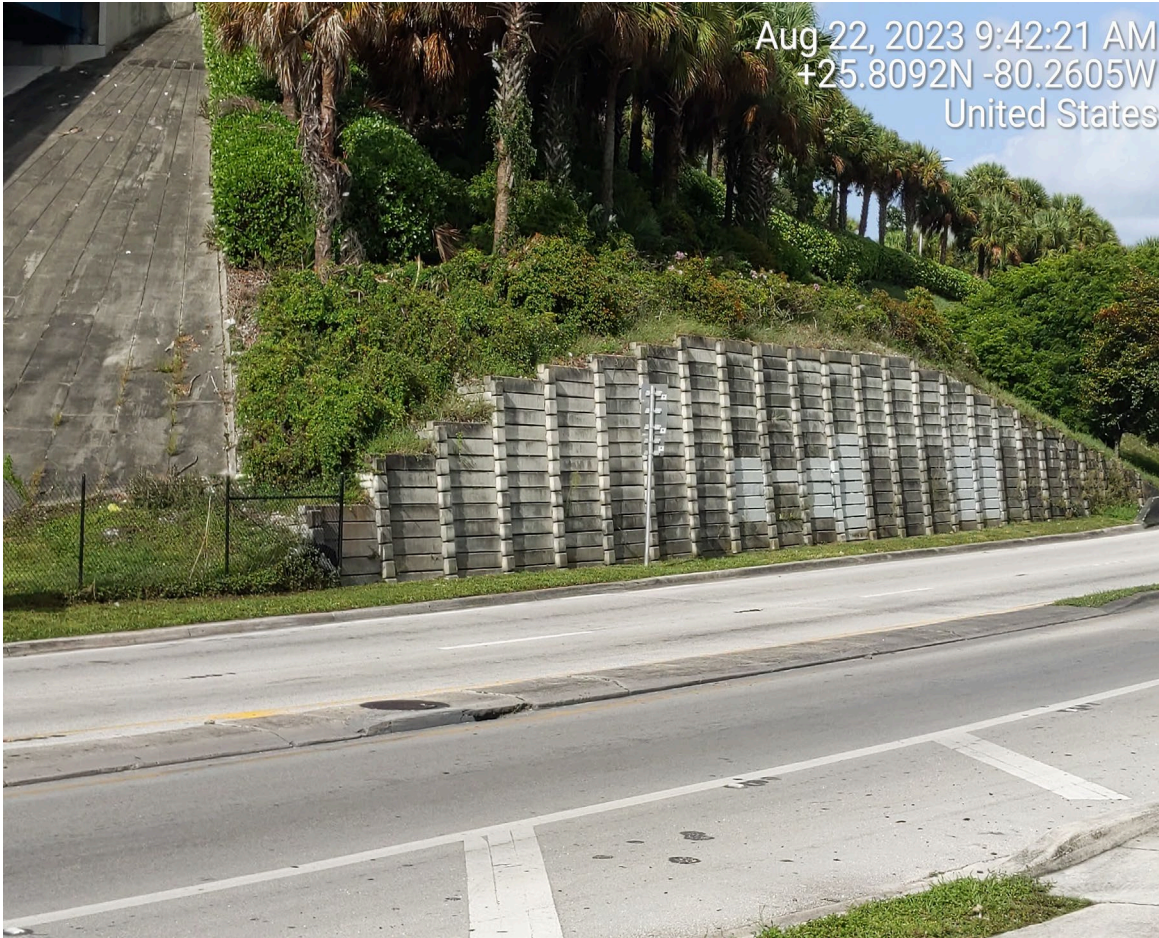
DETERIORATED CLASS V COATING ON RETAINING WALL
