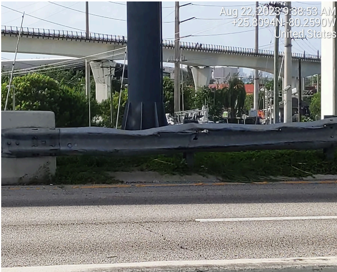
DAMAGED GUARDRAIL
