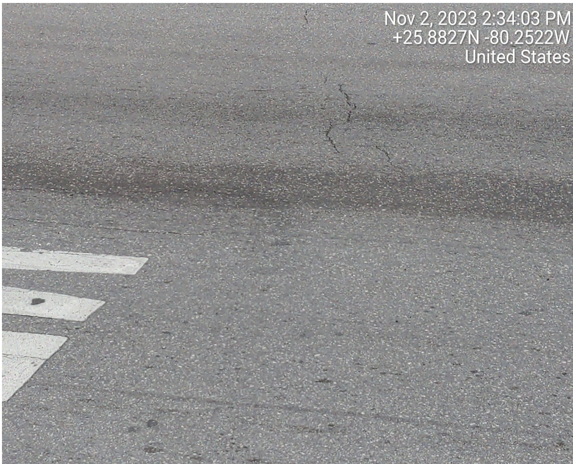
PAVEMENT SETTLEMENT AT PIPE CROSSING
