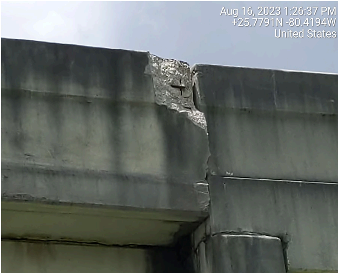
SPALL ON BRIDGE RAILING BRIDGE NO. 871006
