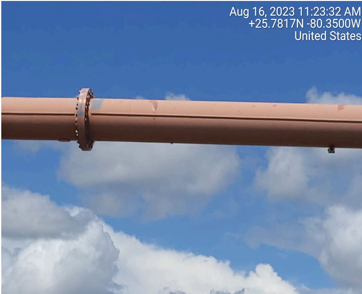
DETERIORATED PAINT ON MONOTUBE (STRUCTURE #875829)
