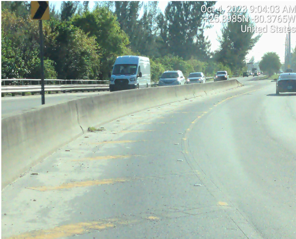
DETERIORATED STRIPING
