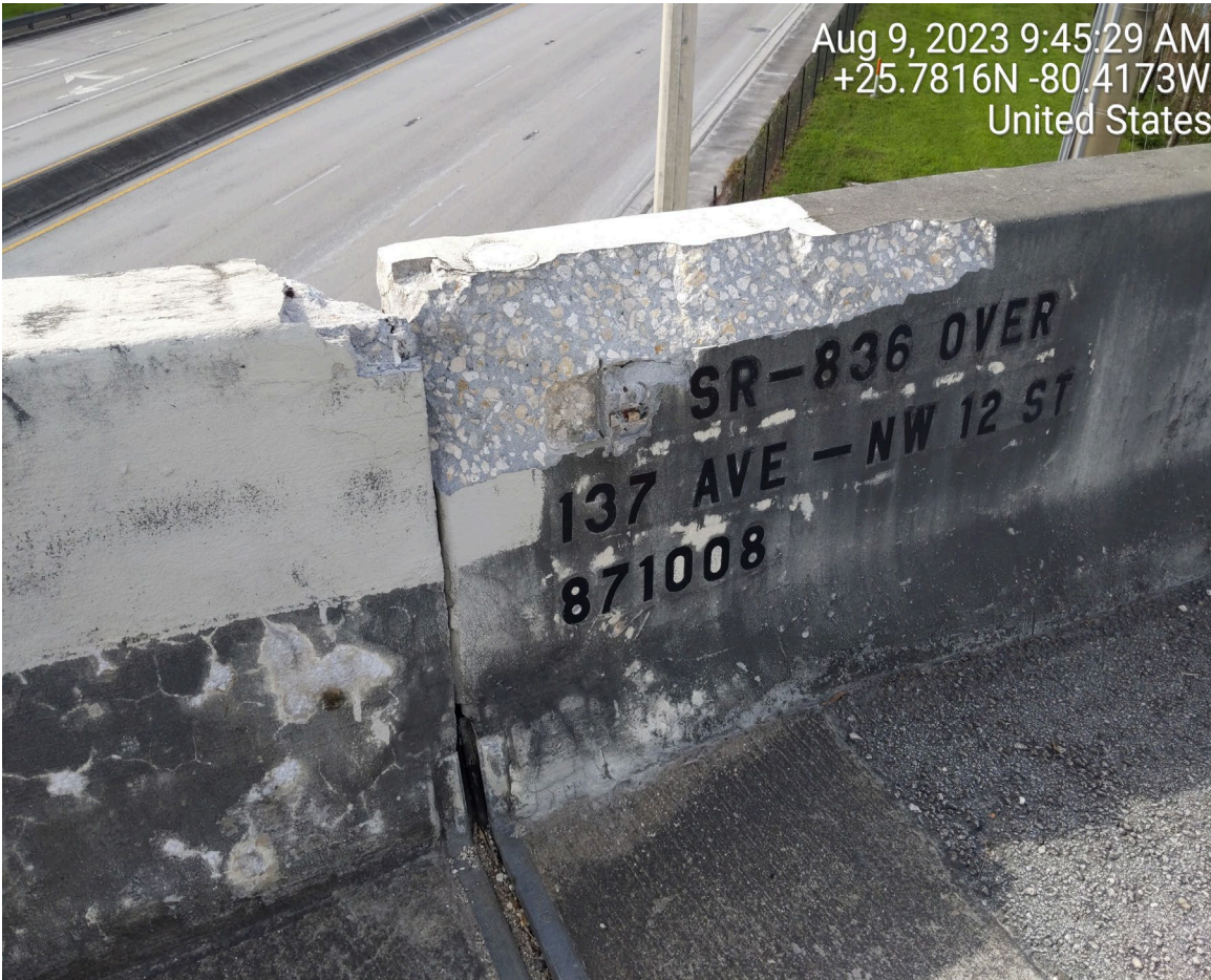
SPALL ON TRAFFIC RAILING (ABUTMENT 1, BRIDGE No. 871008)
