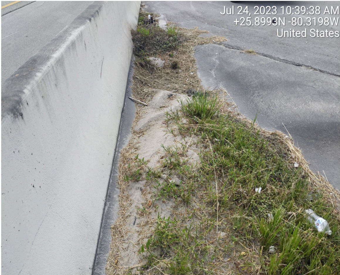
SEDIMENT OBSTRUCTING FLOW ON CONCRETE PLUME
