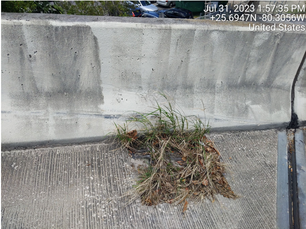
SILTED DECK DRAINS (TYPICAL AT VARIOUS LOCATIONS)
