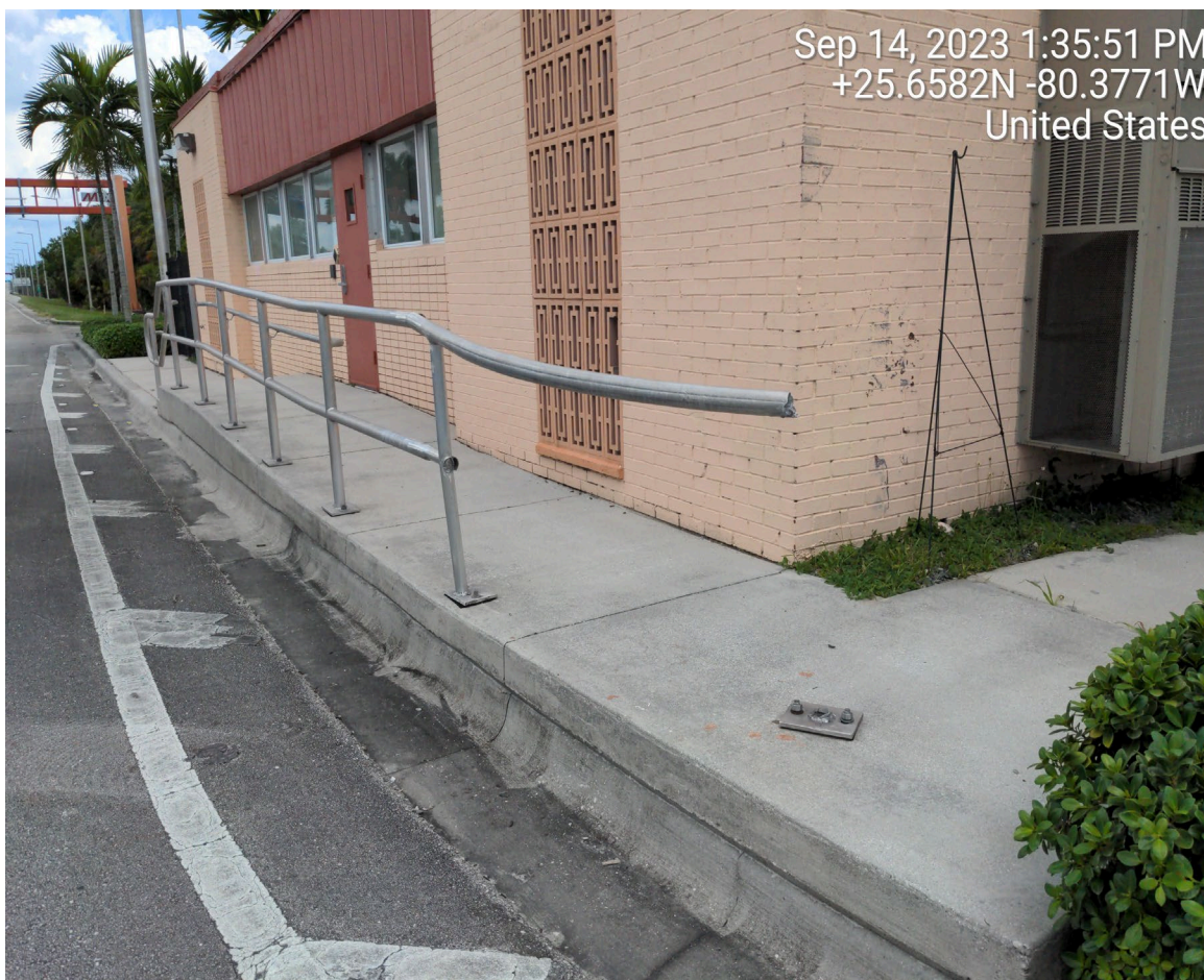
DAMAGED PEDESTRIAN RAILING
