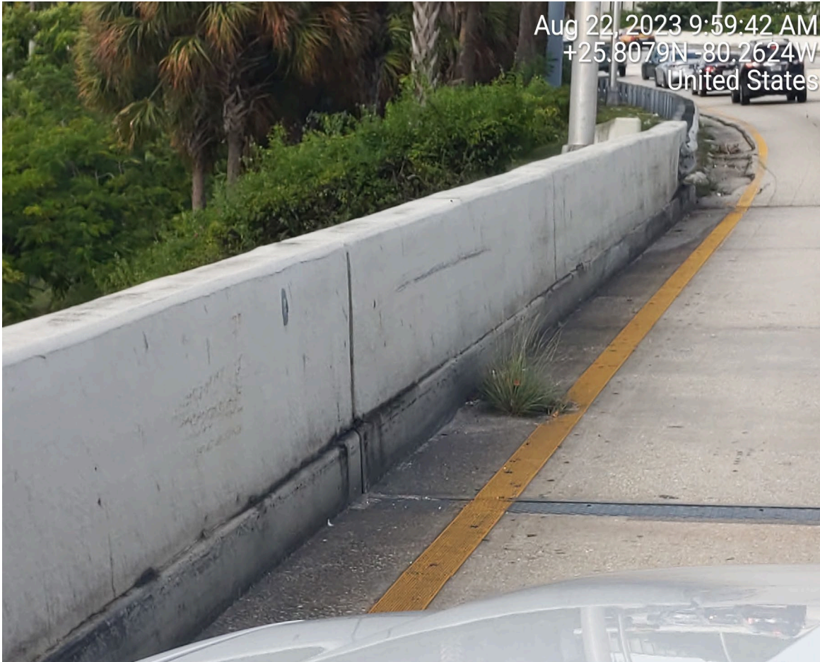
SILTED BRIDGE DECK DRAINAGE INLET
